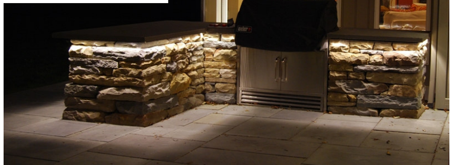
Outdoor Grill Station - Tara Standard Hardscape Fixture in Warm White
